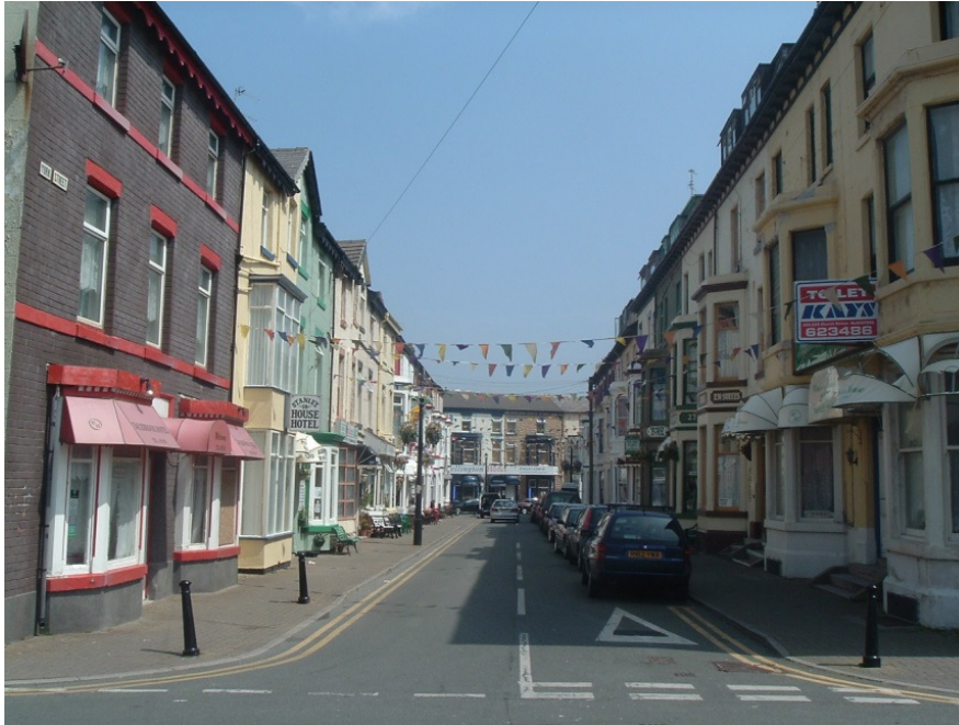
Modern fixed blinds on historic buildings
