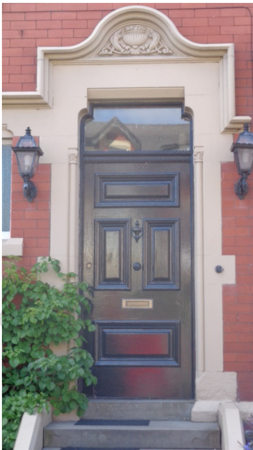
Original late Victorian panelled front door
