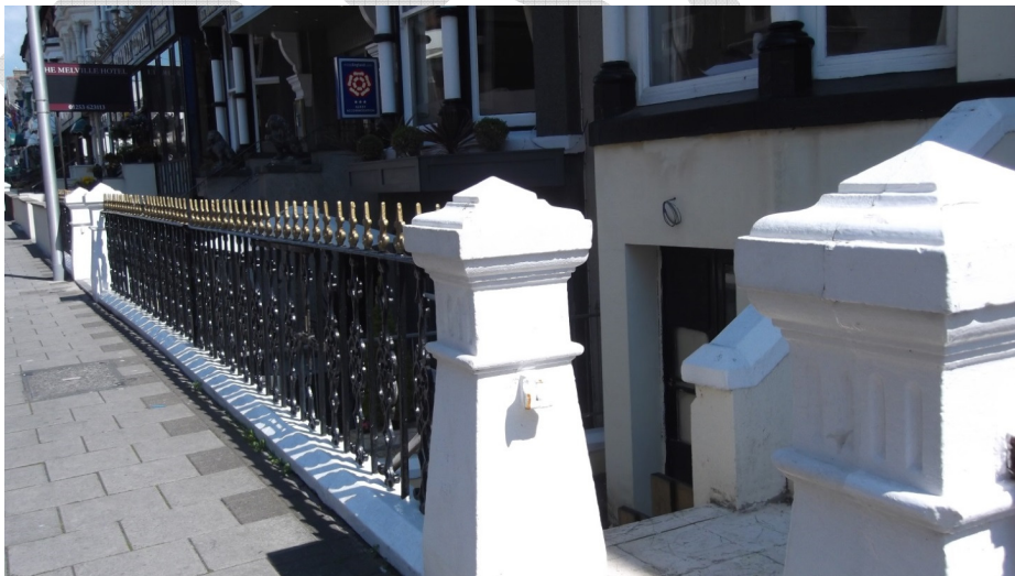
Wrought iron railings on Adelaide Street
