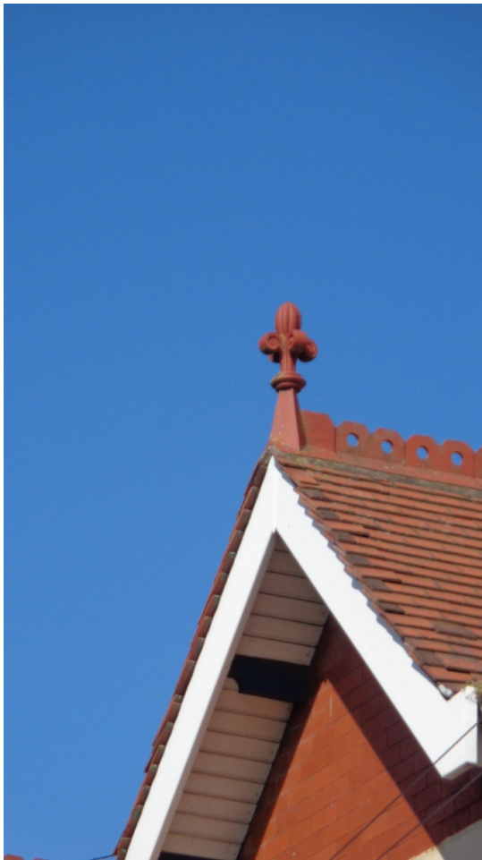
Terracotta finial and ridge cresting
