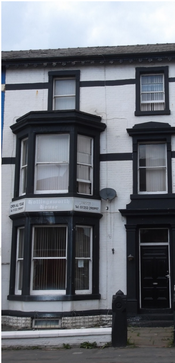
Guest house with original sliding sashes
