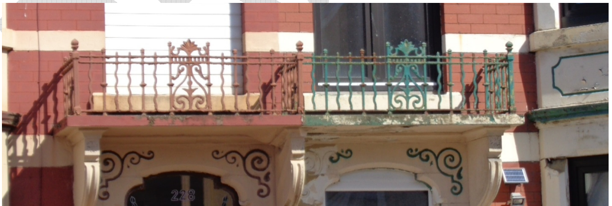
Wrought iron balcony railings
