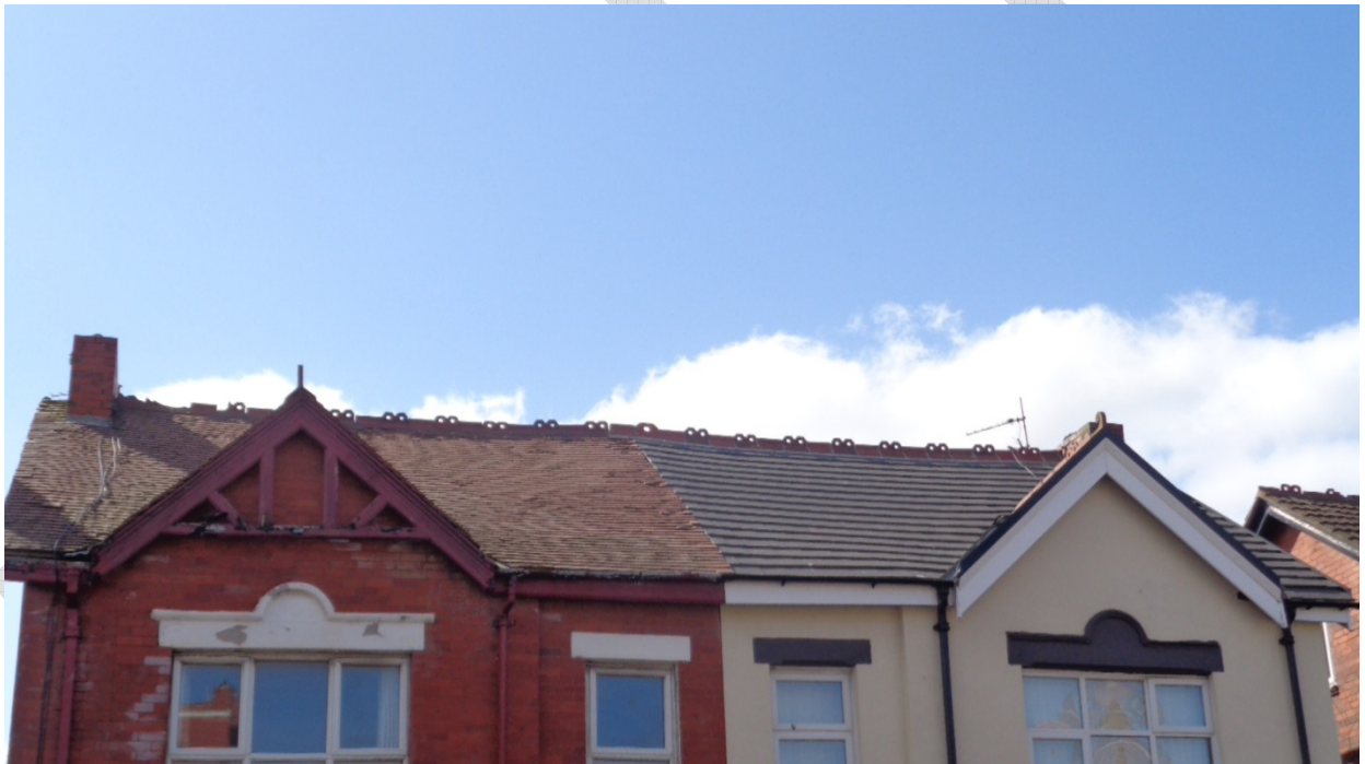
Red clay tile roof covering to the left and modern roof tile to the right of this pair of semi-detached villas
