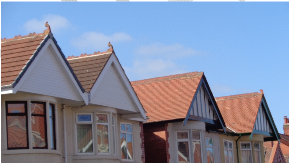
Original half-timbered gables to the right, upvc clad gables to the left
