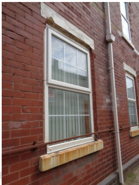
Upvc window frame with 'stick on' glazing bars and top hung upper window
